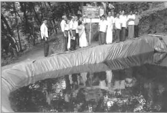
Water harvesting storage tank inaugurated under FPARP project at Vallikadavu
